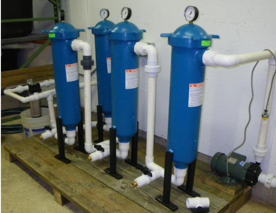
**Figure 2. New filtration system, CAC, Marion State Fish Hatchery.**
