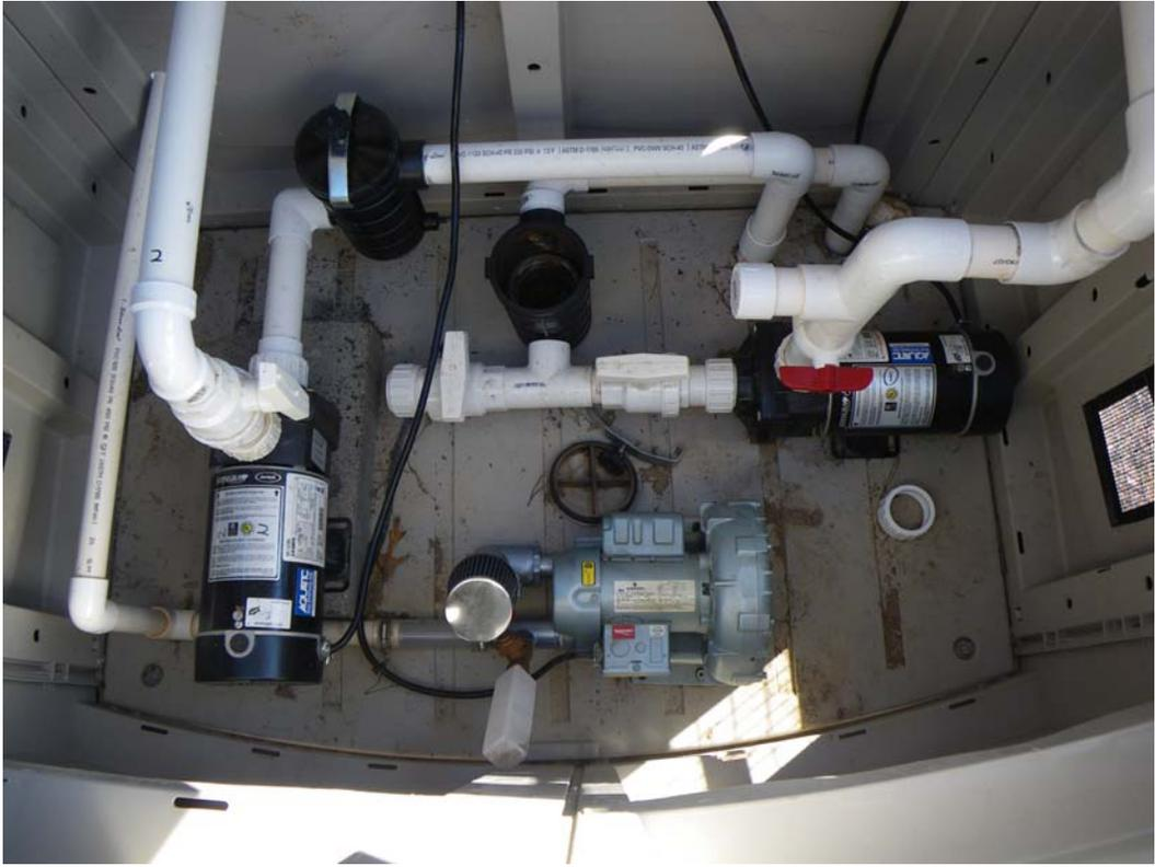
**Figure 6.** Primary system water and air pumps.
