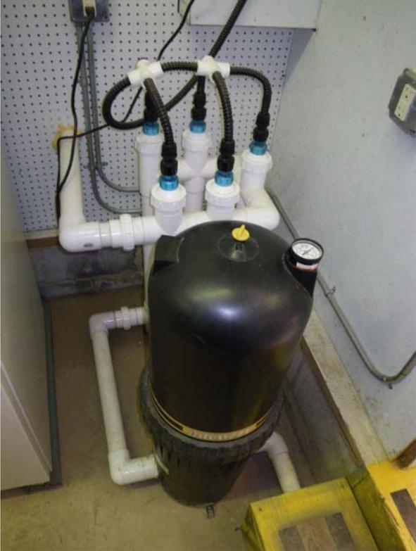
**Figure 7.** Filter and ultraviolet sterilization array on out-going water line.
